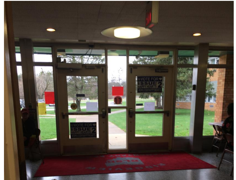
Building lacks a secure vestibule
